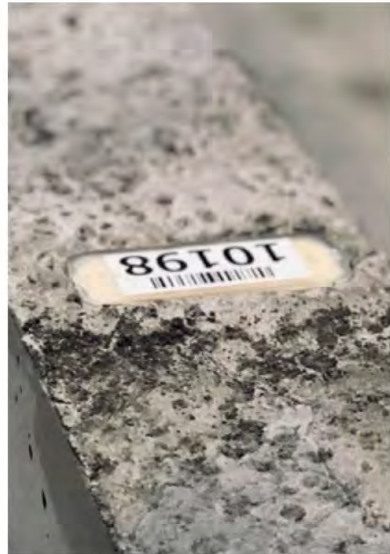
In-situ product information the dormant chip links to information when activated
